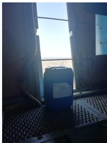
Close-up of the area where the incident occurred, showing the jerry can dimensions with respect to the lower handrail.
