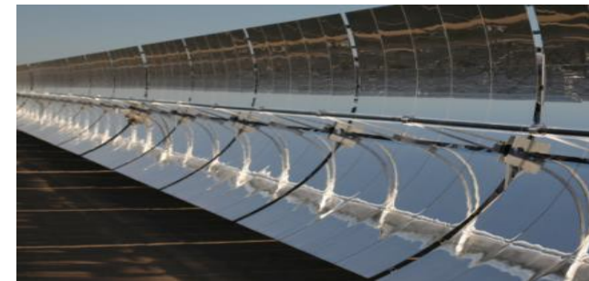
CSP: Nevada Solar One commissioning
