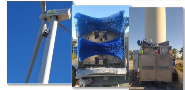
Wind tower cleaning
